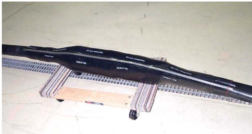
Figure 1 - Cable Joint before Water Housing Installation
