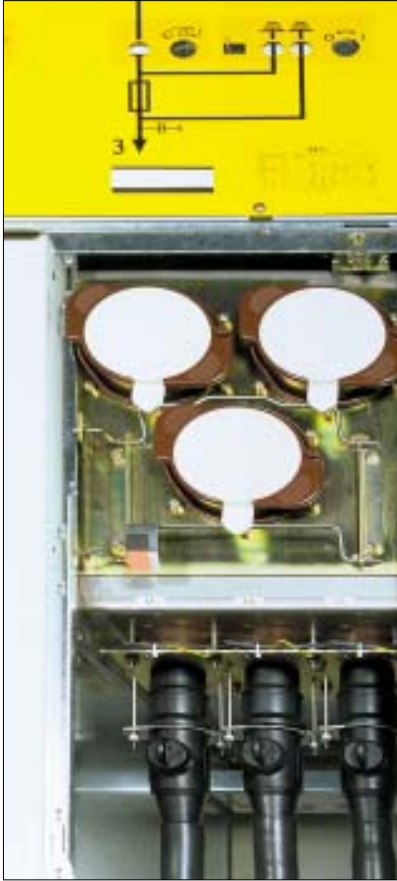
Screened Straight Adaptors installed on SF 6 -switchgear.
